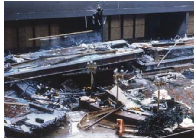
Aftermath of Hyatt walkway collapse.
