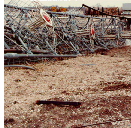
Final (doomed) antenna (“basket”) section of Missouri City antenna.
